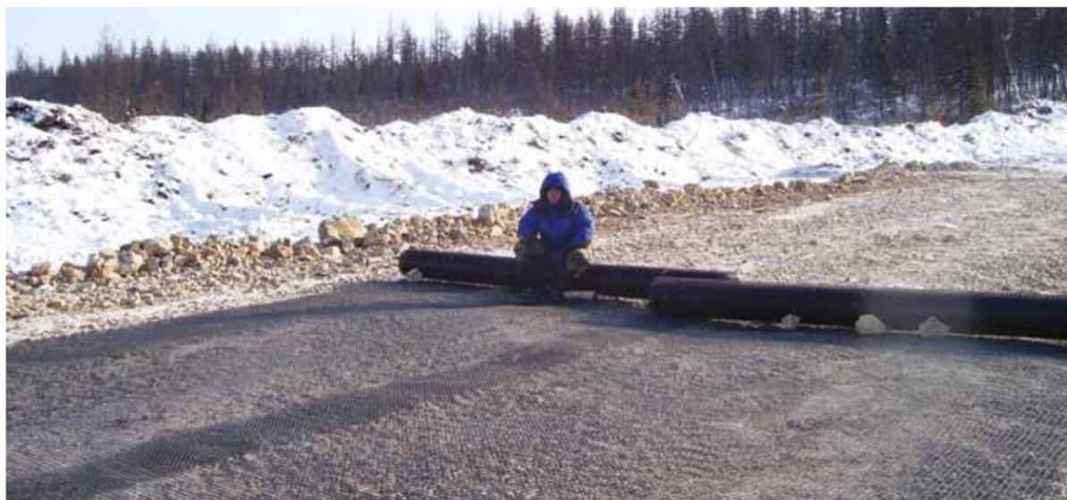
*Tensar geogrids enable significant savings in granular thickness and consequent reduction in construction CO<sub>2</sub> emissions.*
