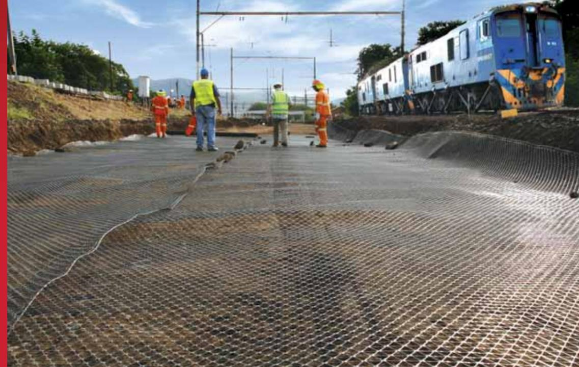
Mechanical stabilisation of sub-ballast can reduce construction costs.
