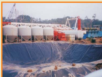
Waste Water Pond, Ramba - Palembang
