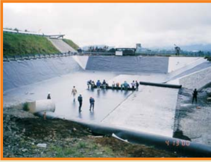
Mud Sump Pond Liner, Pengalengan - Bandung
