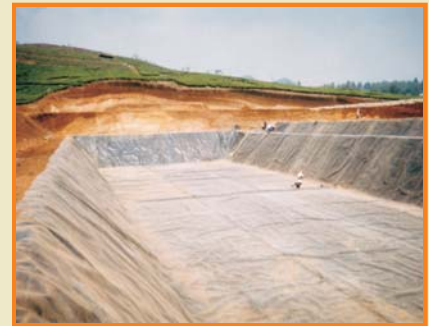
Mud Sump Pond Liner, Pengalengan - Bandung
