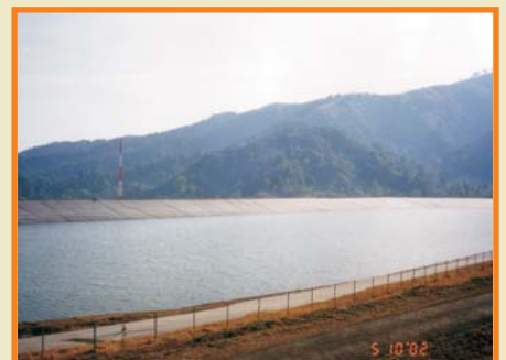
Waste Water Pond - Lombok
